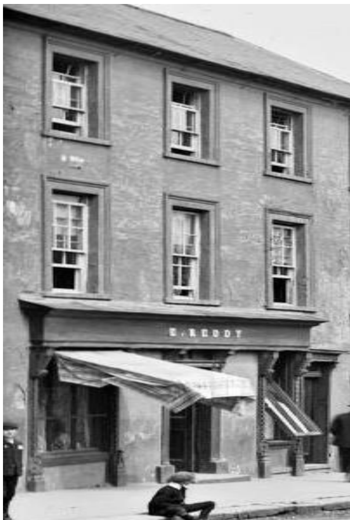
Image of Reddy's shop main street Gorey.
